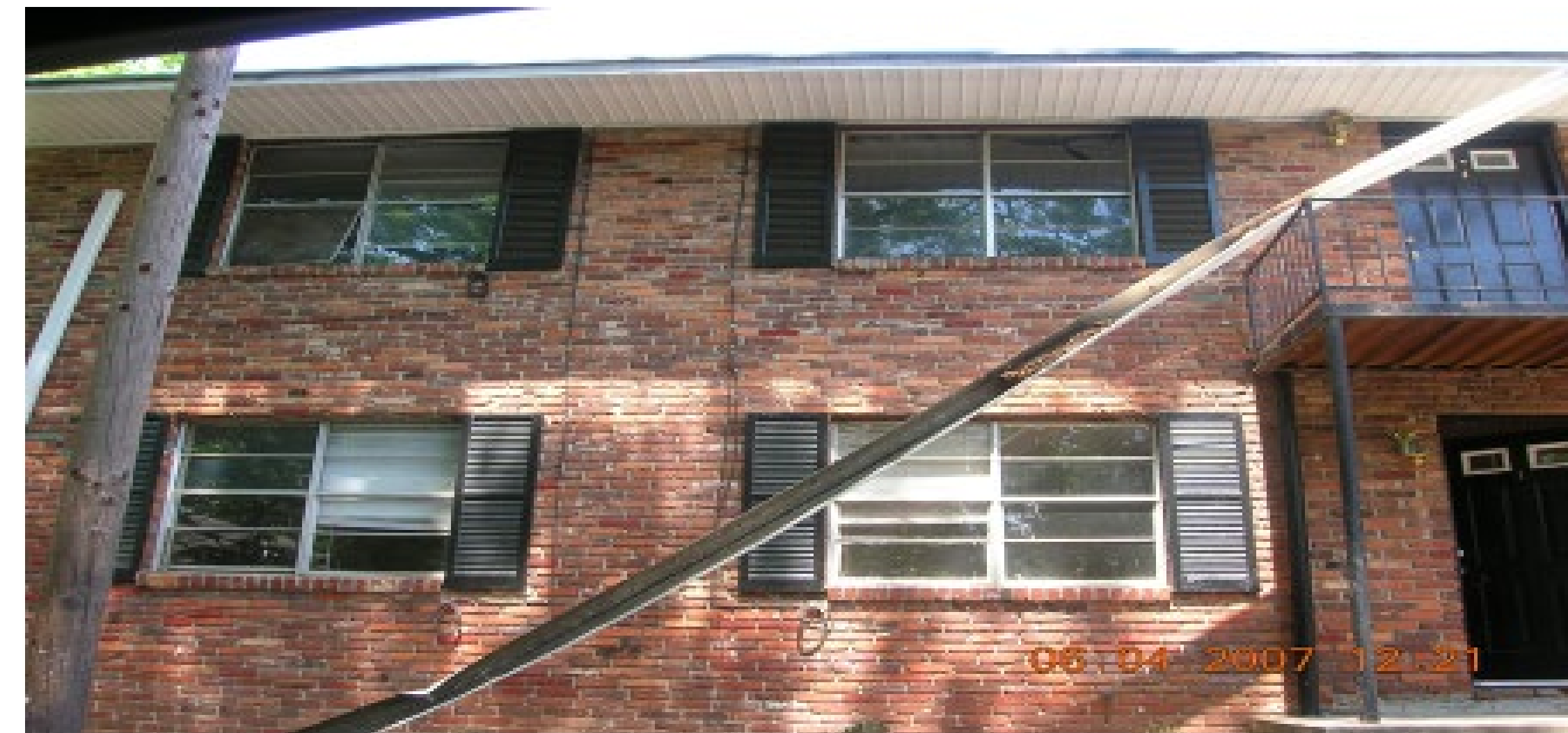
Gutters Hanging Off of Building
