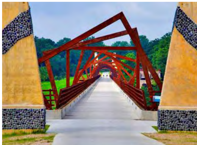
LEFT: The High Trestle Bridge, Woodward, IA
