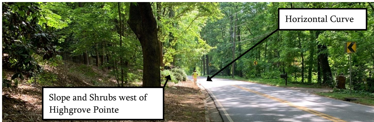
Figure 2: West of Highgrove Pointe; Looking East
