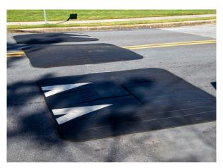
Speed cushions are raised areas in the pavement surface, extending transversely across the travel way in segments, that require vehicles to travel at reduced speeds. Speed cushions can be used along streets with demonstrated speeding problems and few crossing intersections. Speed cushions are similar to speed humps, but they are spaced to allow fire vehicles to straddle the cushions. This has less impact on response time than speed humps.
