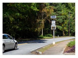
These are highly visible, but have limited effectiveness, with an estimated 4 mph reduction in average speed. Ongoing maintenance is required. The cost of a RSFS in 2020, is approximately \$8,000, including materials and labor.
