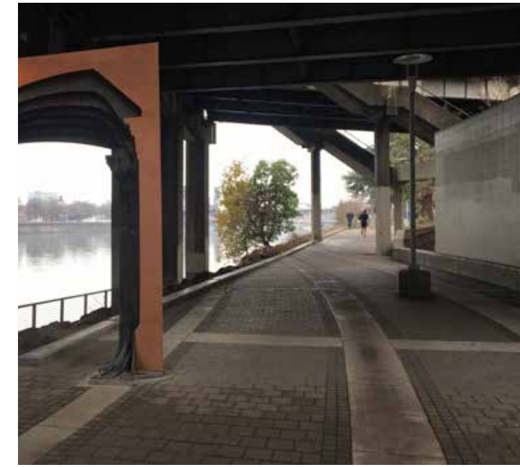
6 Trail Underpass beneath Bridge
