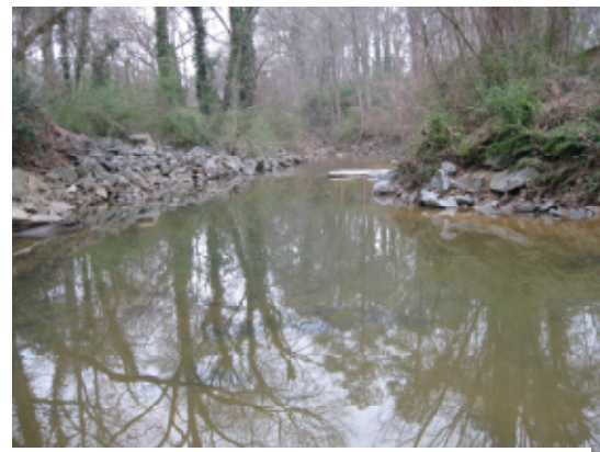
Example of a channel rip-rap lined along the entire bank
