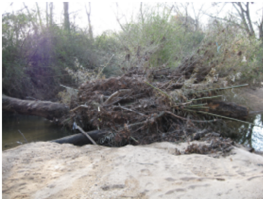
Example of a debris dam observed throughout
