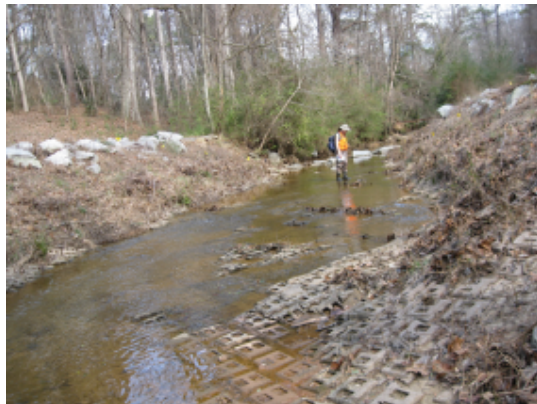
Riprap lined banks were the most common man-made alteration observed
