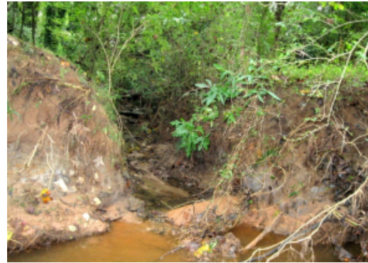
A tributary incised to match bed elevation of main stream
