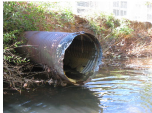
Stormwater outfall on Marsh Creek near 550 Abernathy Road
