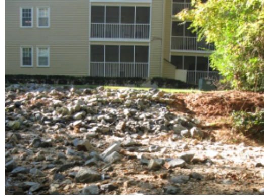
Impervious surface and structure encroachment was second-most common buffer encroachment observed
