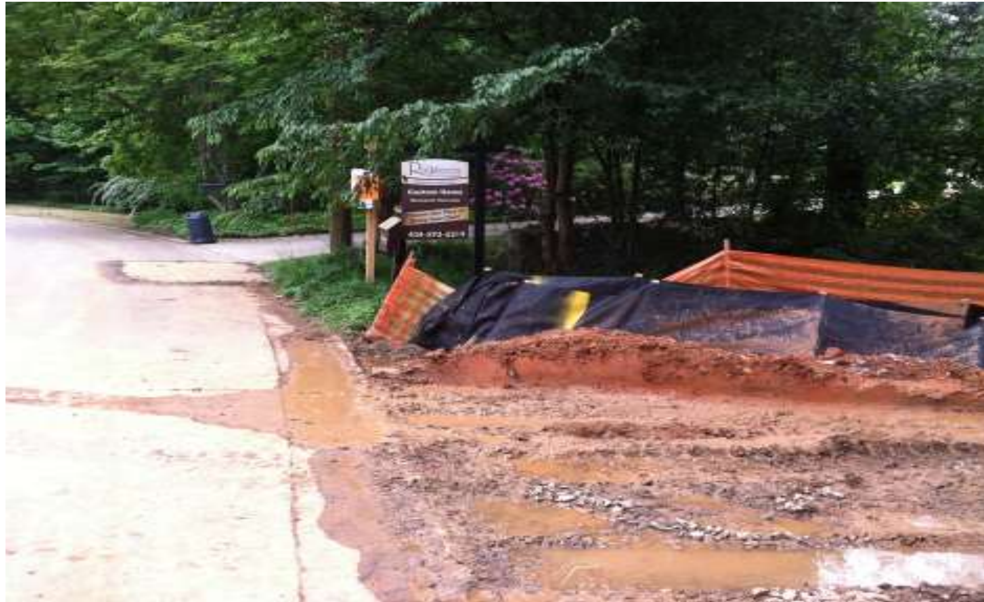
Illegal Construction Exit
