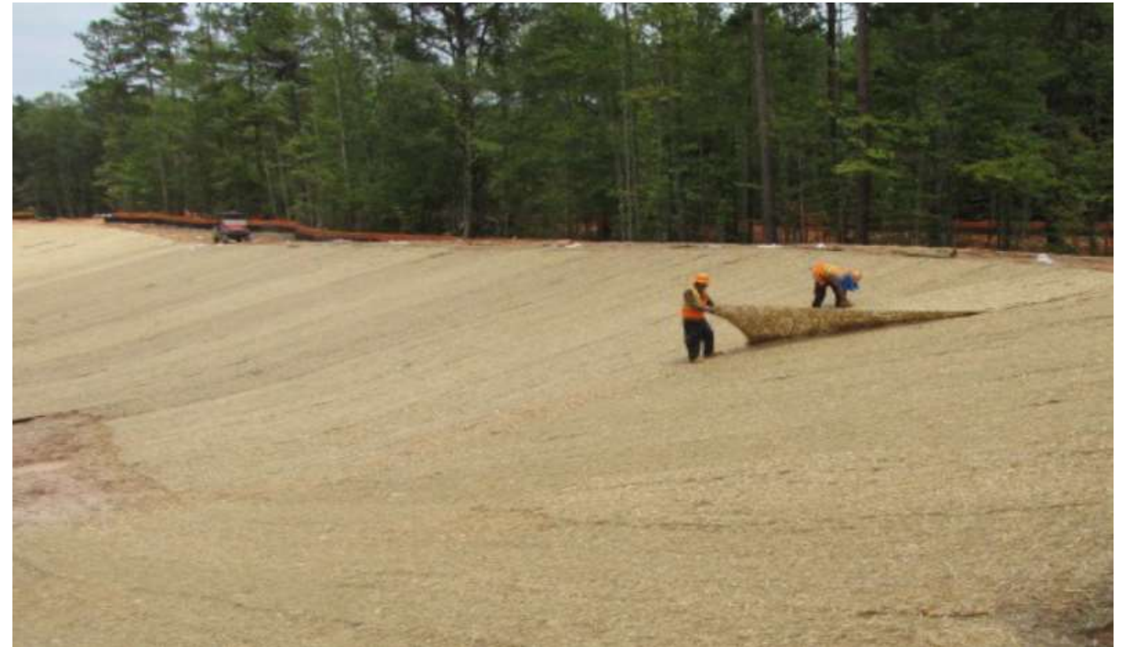
Slope Stabilization With Seeded Mats
