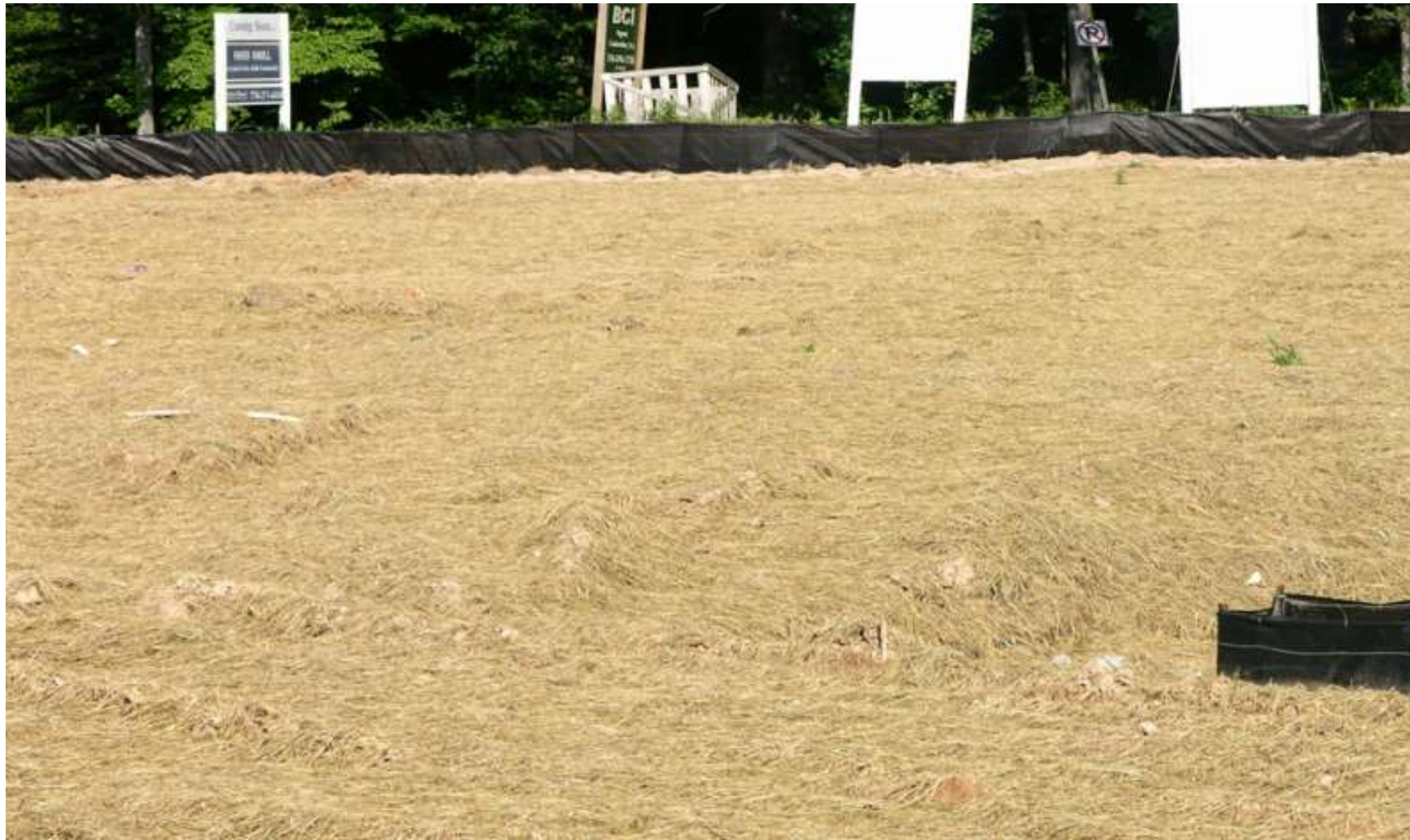
Mulching – Minimum 90% Coverage
