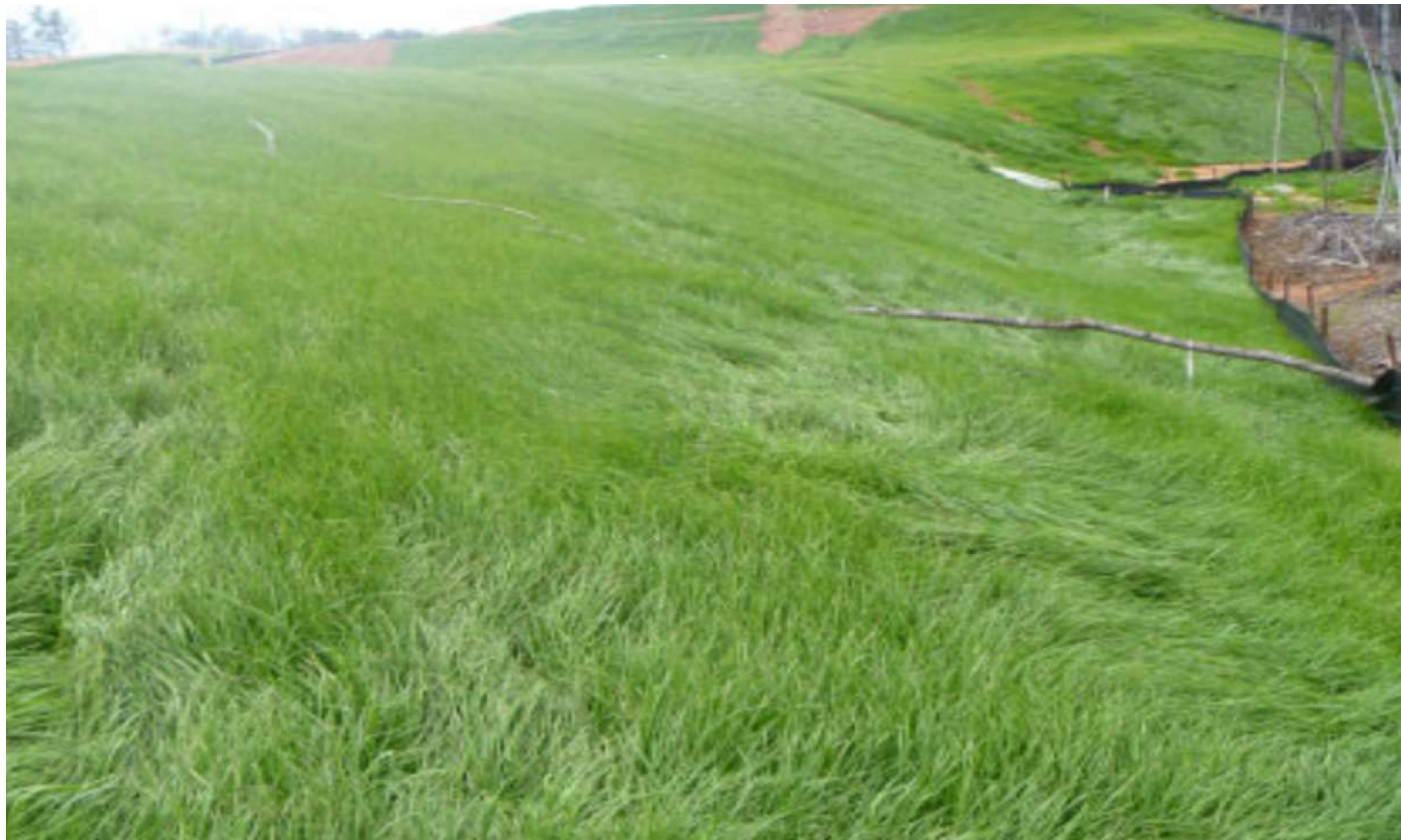
Temporary Seeding: Minimum 70% Germination
