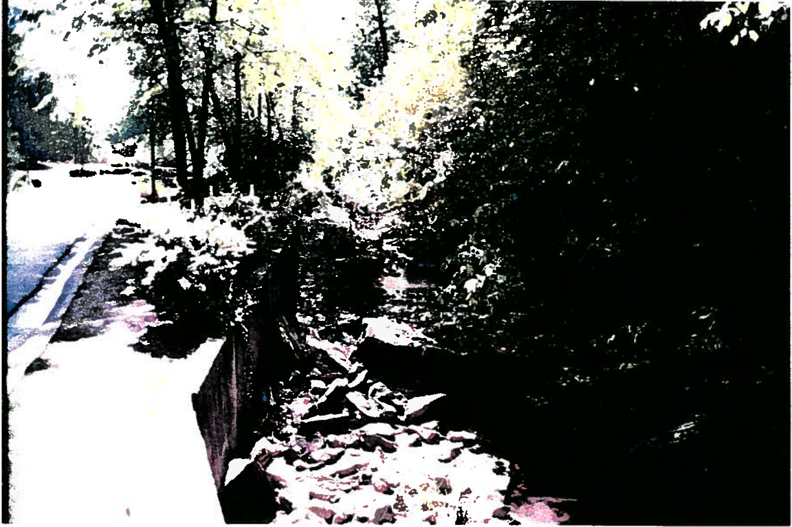
PHOTO 19 - REPRESENTATIVE VIEW OF SS-7, POWERS BRANCH (Note pipe and retaining wall in creek and adjacent roadway.)
