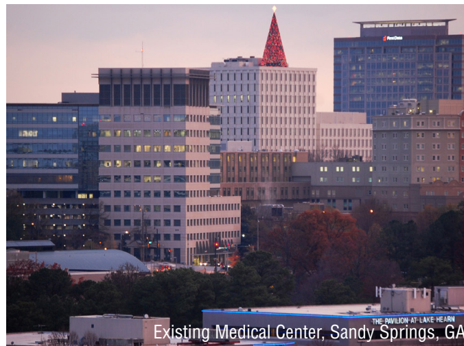
Existing Northside Hospital, Sandy Springs, GA
