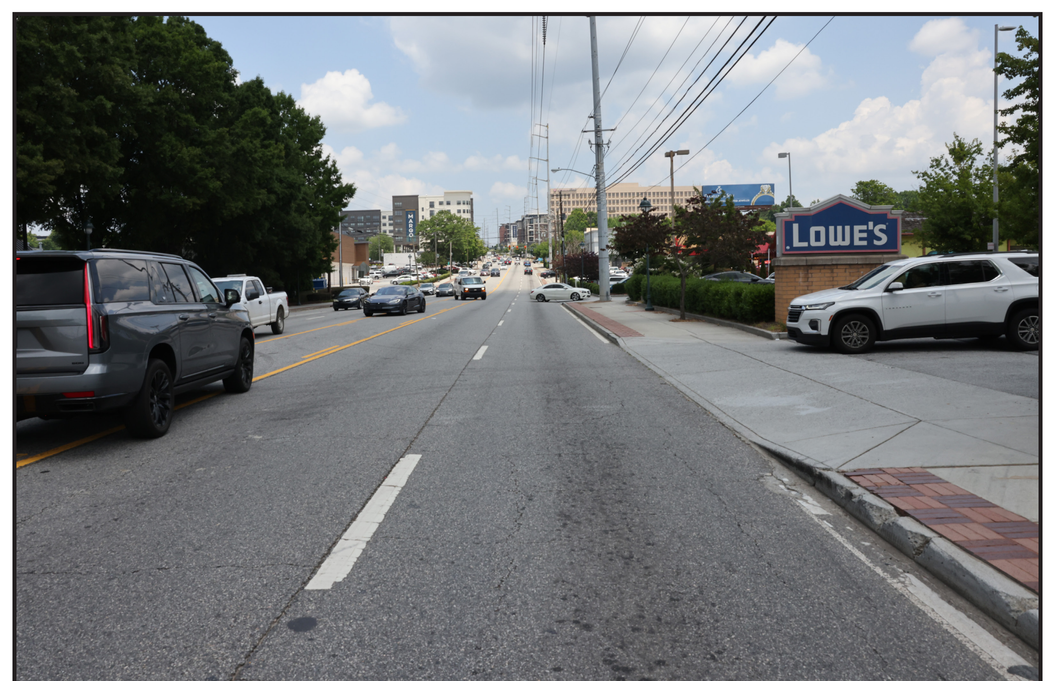
Roswell Road between Hammond Drive and Cliftwood Drive/Carpenter Drive experienced a high concentration of crashes, many of which were associated with left-turn movements into and out of driveways. Of the 215 crashes in this area, 60 occurred at driveways. The installation of a median will help reduce crashes along this section of Roswell Road.
