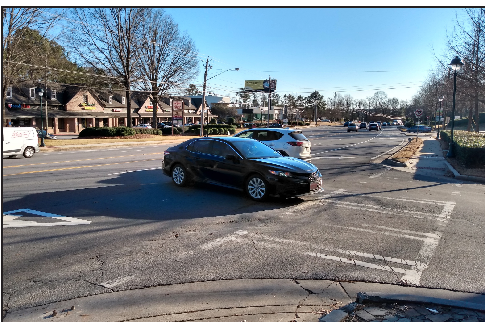
The driveway at the Quik-Trip gas station south of Grogans Ferry Road was the site of multiple left-turn and driveway-related crashes, including one fatal crash. This location is part of the Roswell Road/Grogans Ferry Road Intersection Improvement Project, which will include median installation.
