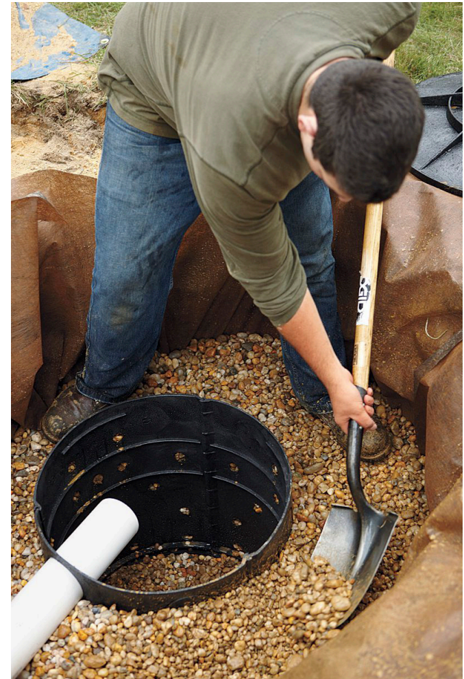
Figure 11 | Drywell installation
