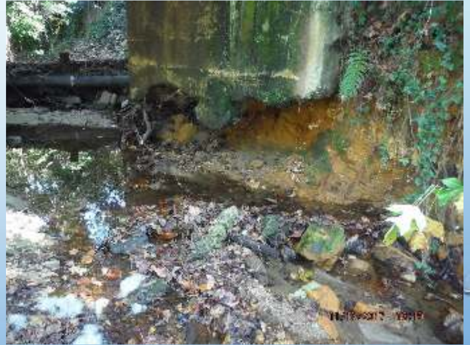
Eroded Infrastructure Support near Hunters Branch Drive (Private Property) Marsh Creek
