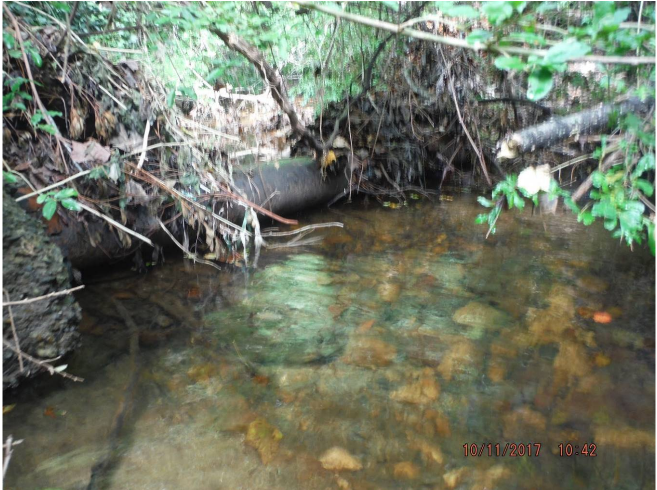
Figure 3-6 Debris Dam along the tributary in Subwatershed NC10 (MP#1011)
