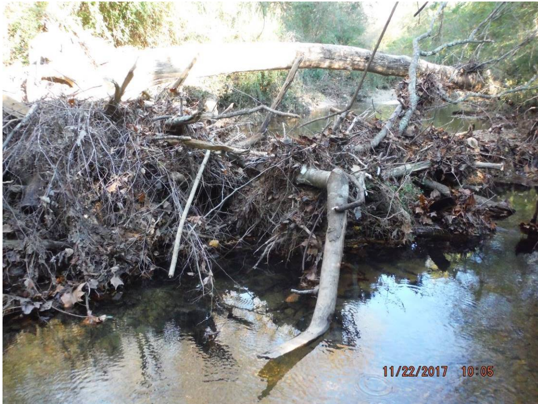
Figure 3-26 Debris Dam in Subwatershed LI01 (MP#1091)
