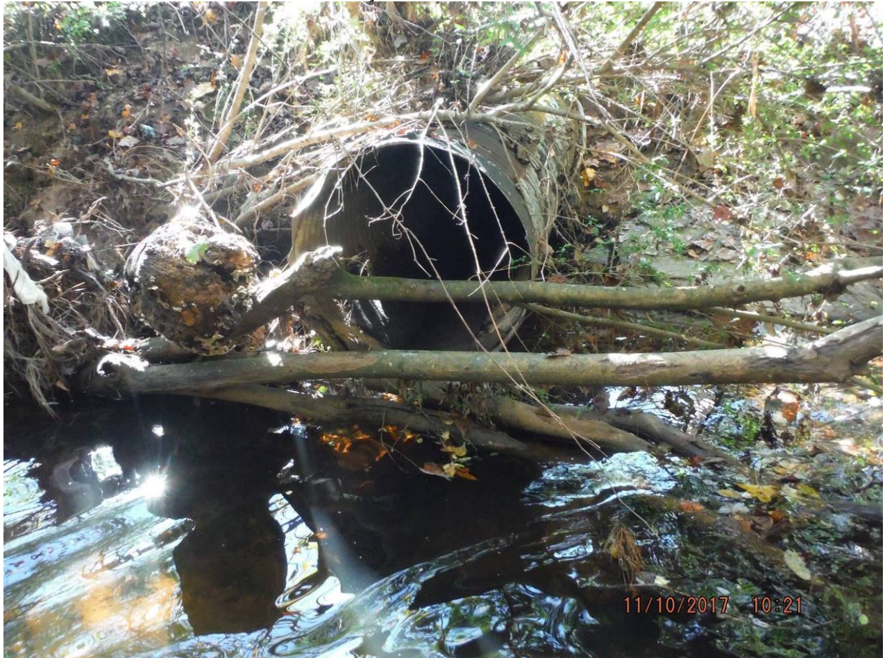
Figure 3-20 Stormwater Outfall in Subwatershed MC05 (MP#1058)
