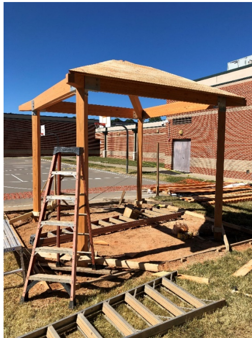
Sandy Springs Charter Middle School Small Pavilion Installation
