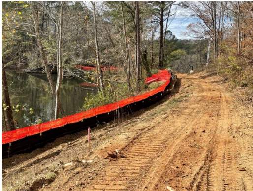
Trail 2A Grading Trail
