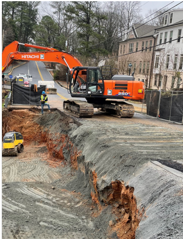
Water Main Break Repairs on Franklin Road
