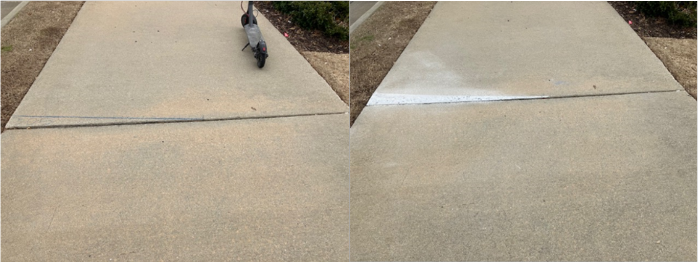
Sidewalk Trip Hazard Repairs
