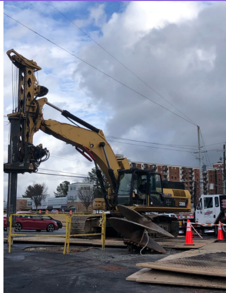
Georgia Power transmission tower foundation work for Project TS-191
