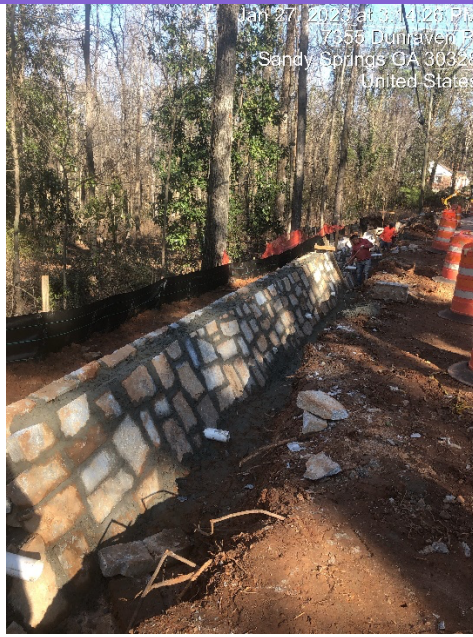
Dalrymple Sidewalk Retaining Wall Construction Continues – TS168
