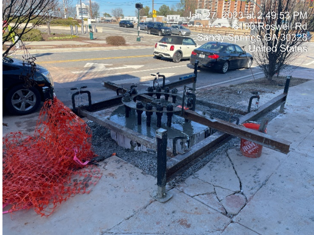
GA Power Transmission Pole Foundation Installation for Project TS-191
