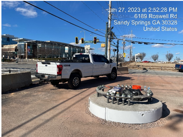
GA Power Transmission Pole Foundation Installation for Project TS-191
