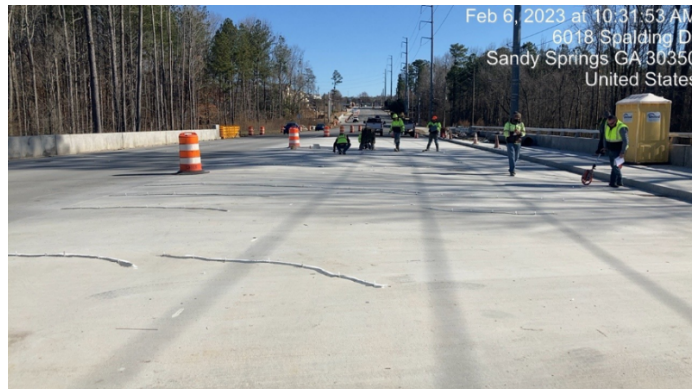
Spalding Drive Improvements bridge deck work underway
