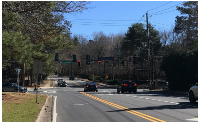
Peachtree Dunwoody at Windsor new signal in operation
