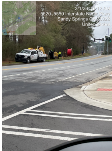
Interstate North Fiber Project installation continues
