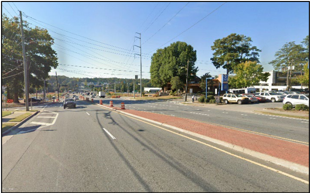
Figure 14. Concrete Median along SR 9 (Roswell Road) in Sandy Springs
