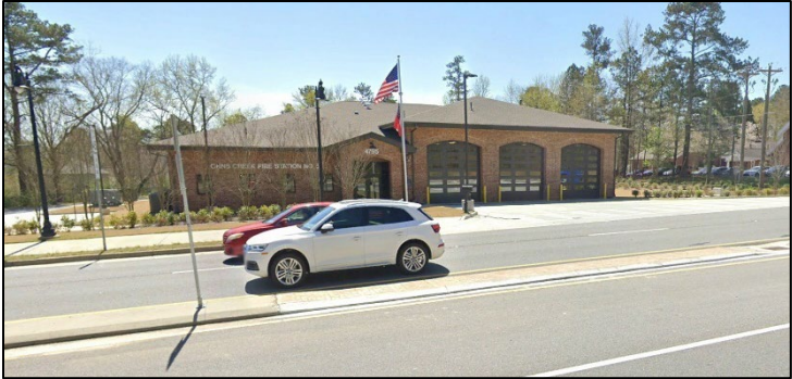
Figure 11. Mountable median adjacent to fire station (Kimball Bridge Rd, Alpharetta, GA)
