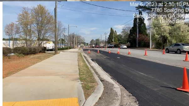
TS-166 Spalding Widening – Milling and Prep for Final Paving Underway
