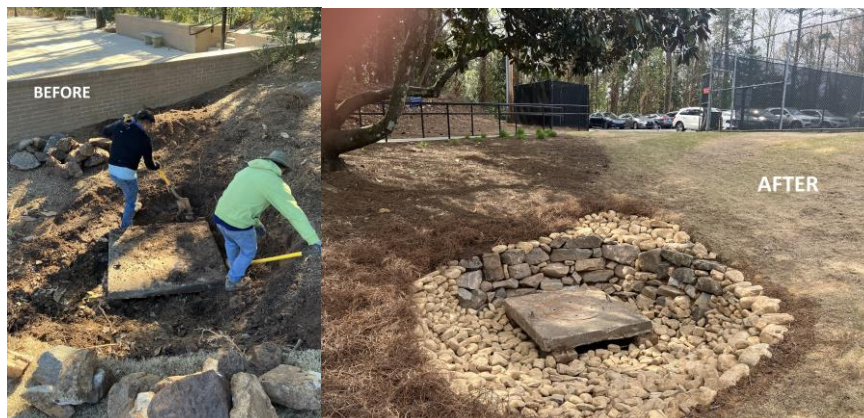
Abernathy Arts Center Drain Repair
