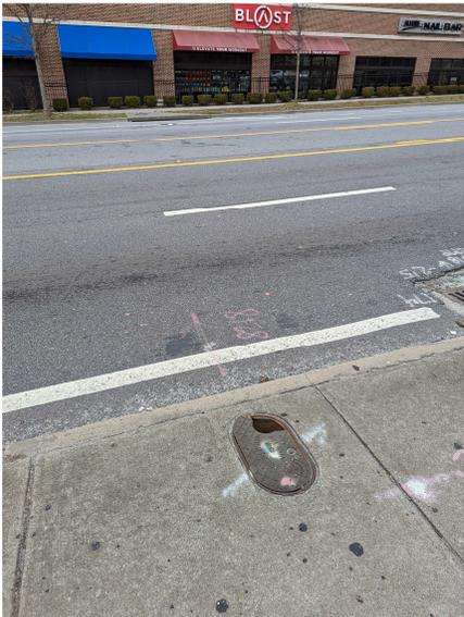
Broken plate in the sidewalk is a tripping hazard for pedestrians.
