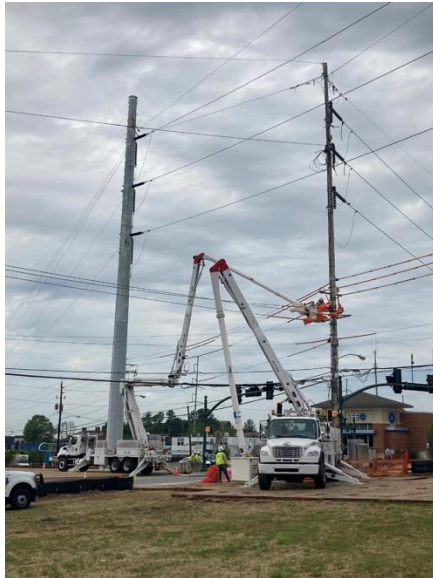
TS-191 Mt. Vernon Highway at Roswell Road Intersection Improvement Project – Georgia Power Company transmission tower installation.
