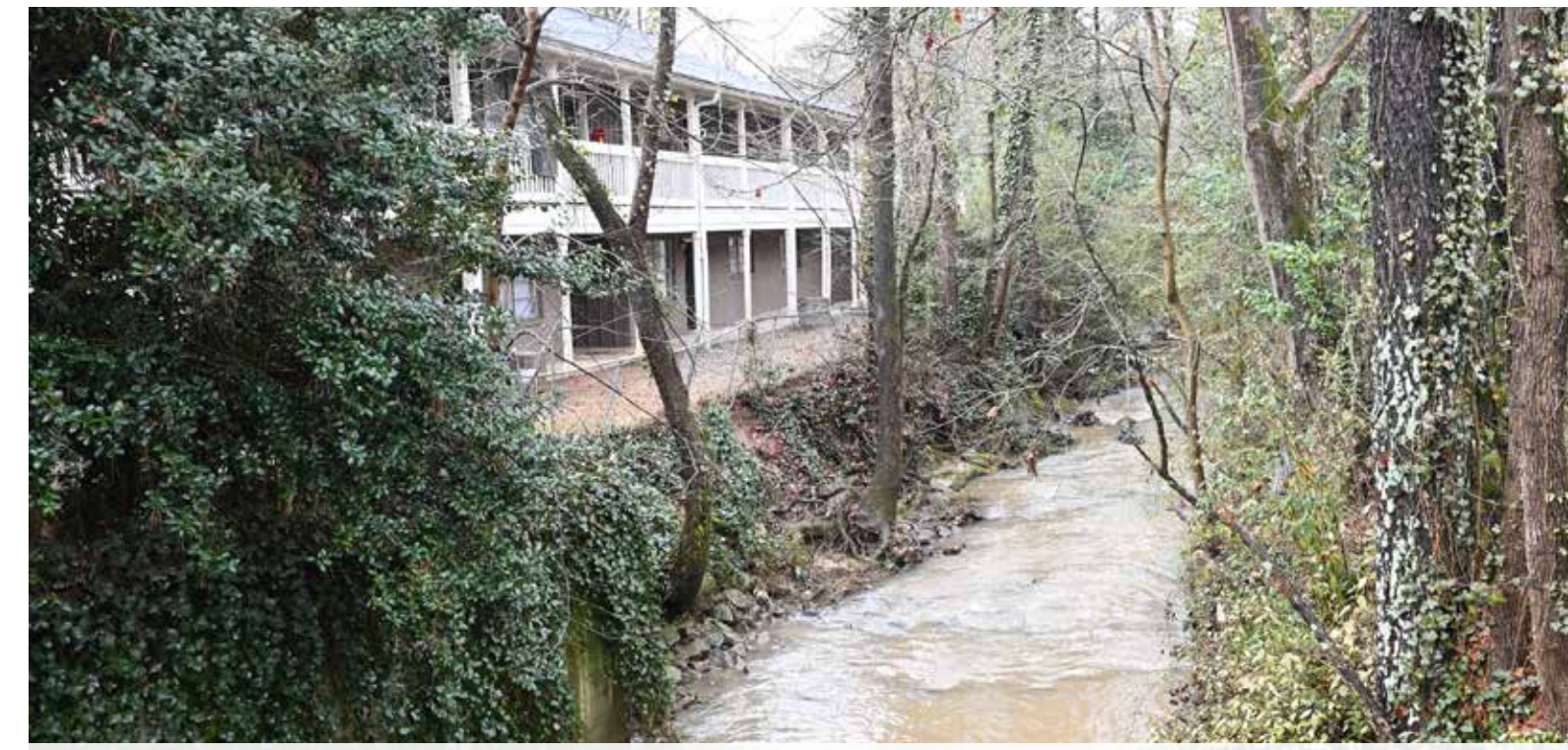
Stream bank conditions along Long Island Creek
