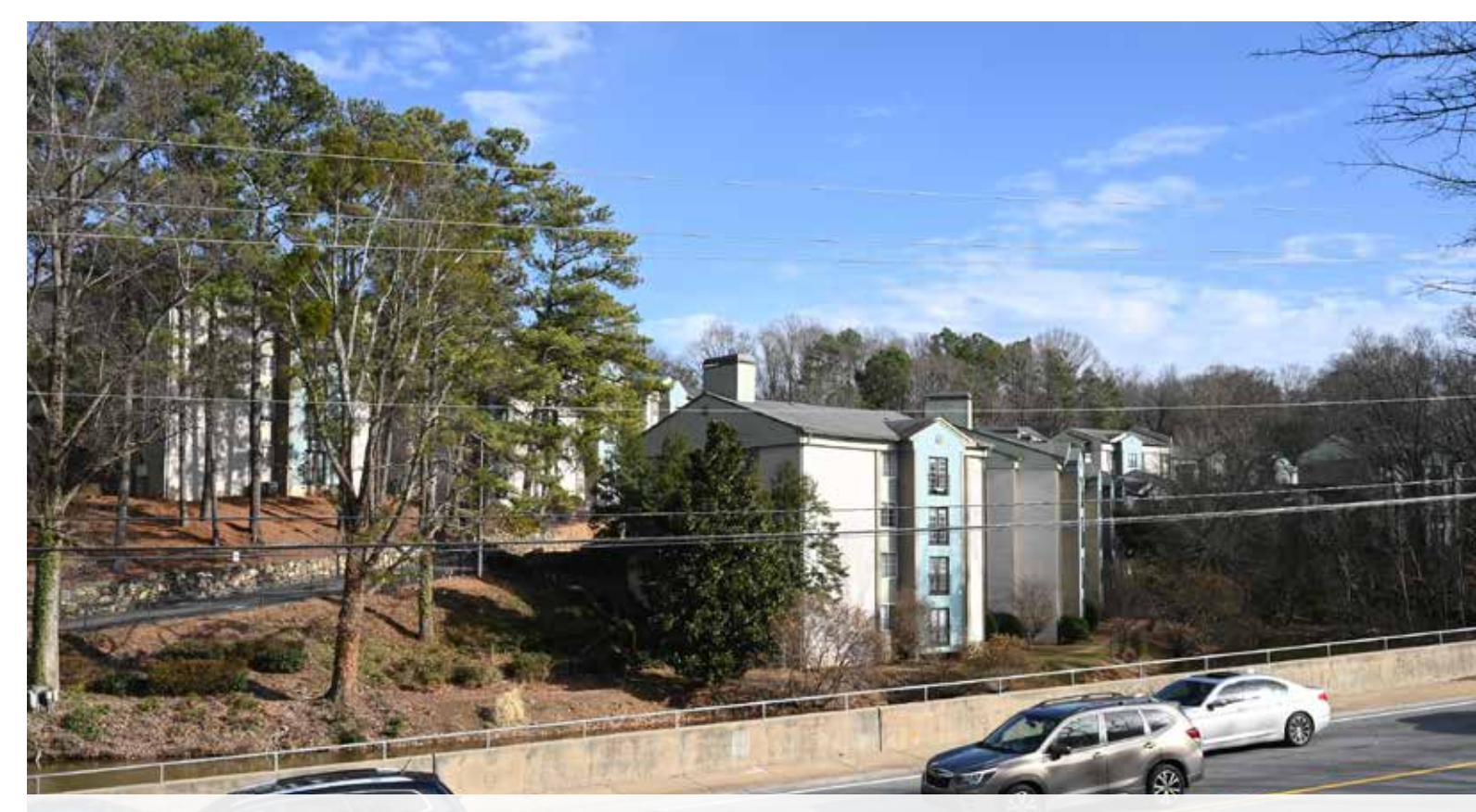
Residential communities with challenging slopes adjoining Roswell Road (on foreground)
