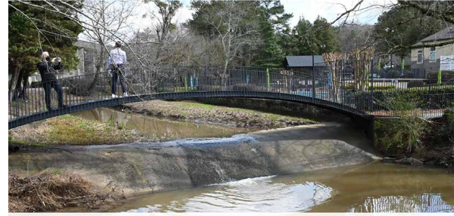
A dam/embankment across Long Island Creek
