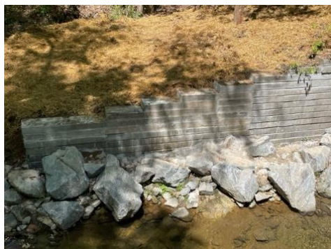
Bridge Maintenance and Repair (left) - bridge wing wall repair and rip rap installation at Riverside Drive over Chattahoochee River Tributary. Bridge Painting (right) - Powers Ferry Road at Long Island Creek
