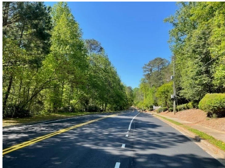
Paving on Roberts Drive (from SR400 bridge to Gettysburg Place)
