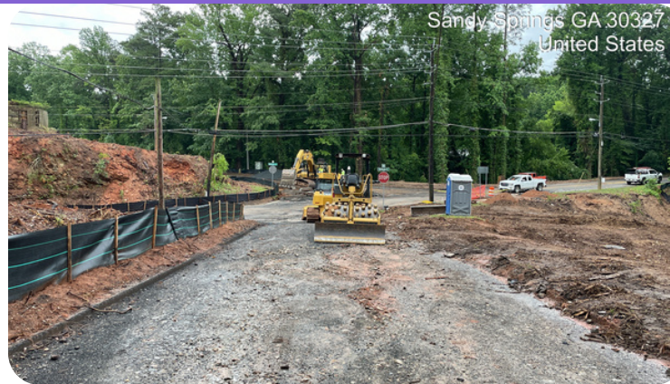
TS106 Northside Drive at Riverview/Old Powers Ferry Road intersection site work
