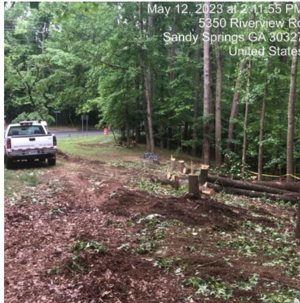
TS-106 Northside at Riverview/Old Powers Roundabout preliminary clearing underway
