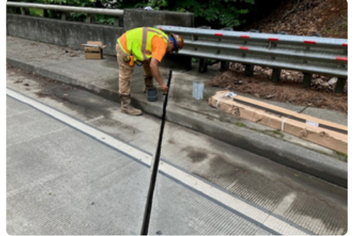
Bridge Maintenance Project Concrete pour at field 2
