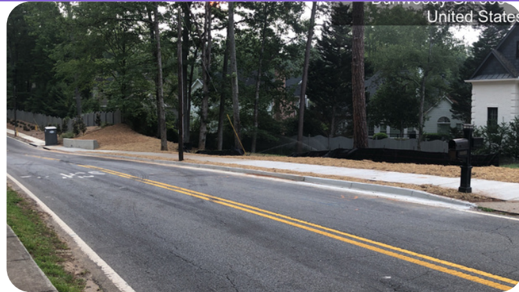
⤴ T6021-1 Spalding Drive sidewalk completed
