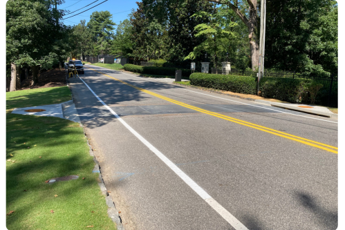
Northside Drive Stormwater Northside Drive Stormwater Infrastructure Rehabilitation
