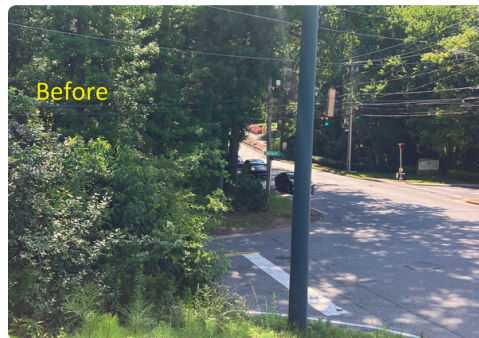
Hammond Drive from Boylston Drive Removing plant material.
