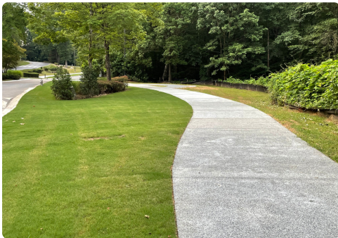
Trail 2A Landscaping progress.
