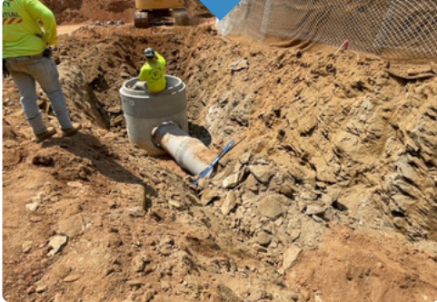
TS106 Northside Drive, Old Powers Ferry Road, Riverview Road Site Work
