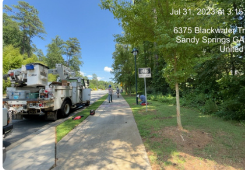
T2307 Johnson Ferry Road Pedestrian Lighting near completion
