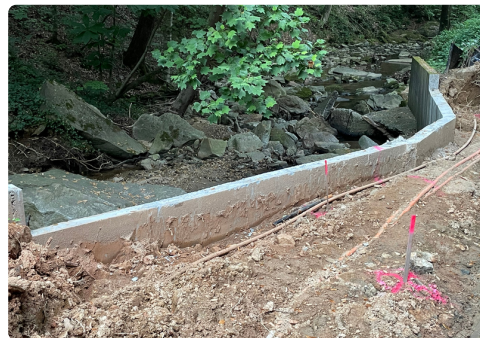
Trail 2A Rubble wall in progress
