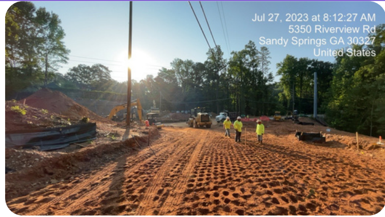
TS106 Old Powers Ferry Road - Riverview Intersection Site Work
