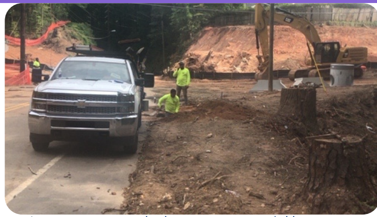
TS106 Northside Drive at Riverview/Old Powers Ferry - Intersection site work.
