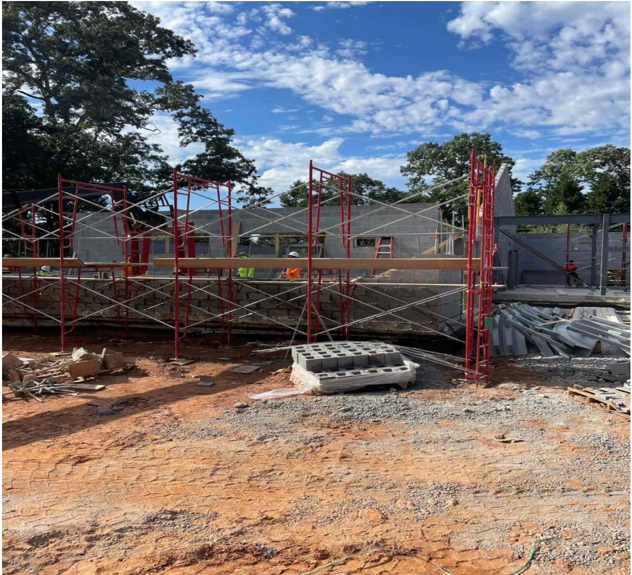
Continuing Installation of Exterior CMU at the Electrical / Generator Rooms
