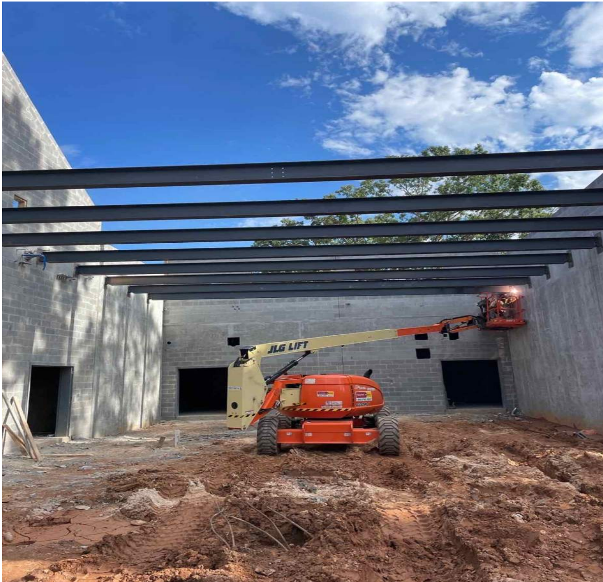
Continuing Structural Steel at Apparatus Bay Roof
