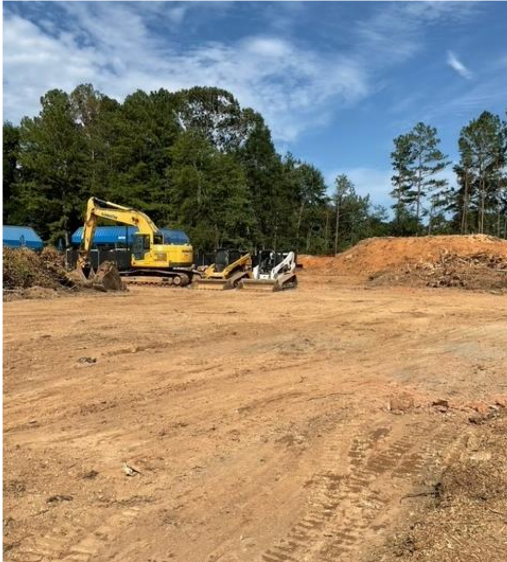
Begin Stripping Topsoil and Grading
