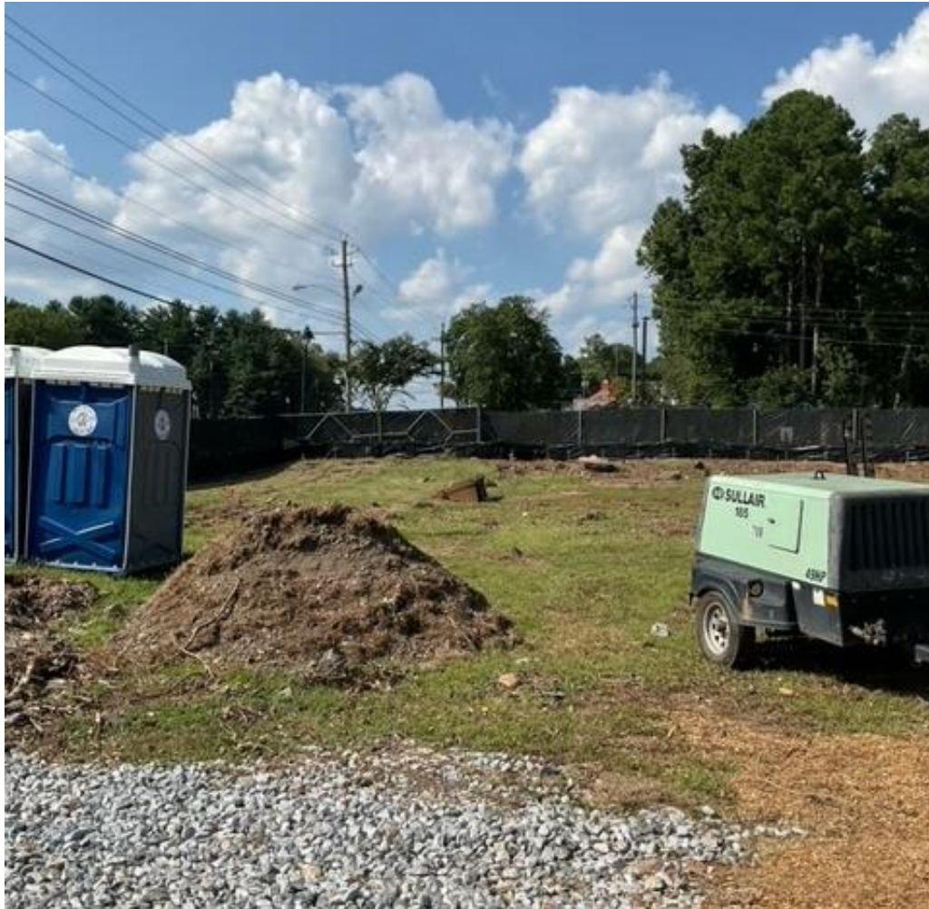
Begin Stripping Topsoil
