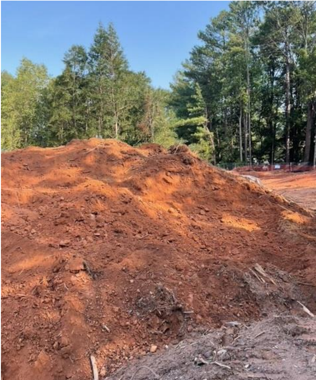
Continued Grading and Export of Unsuitables
