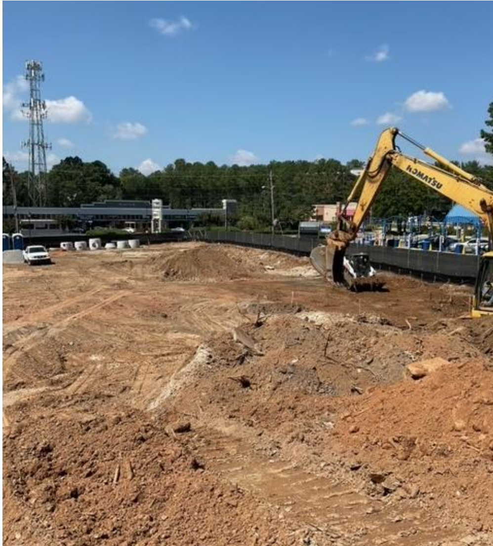
Continued Building Pad Preparations
