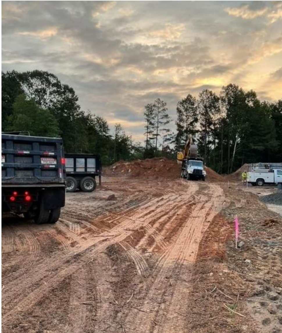
Continued Export of Dirt and Unsuitable Materials
