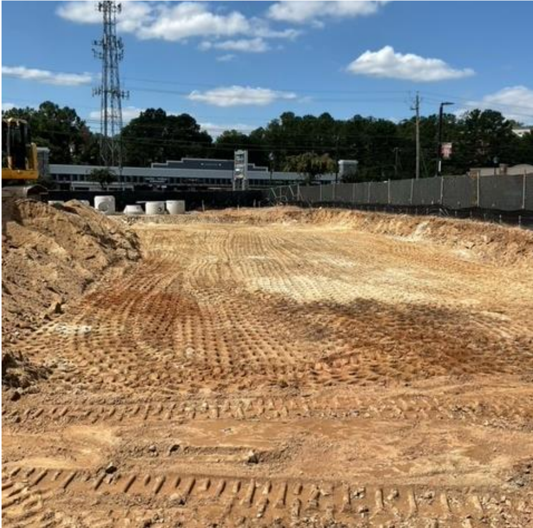
Continued Building Pad Preparations
