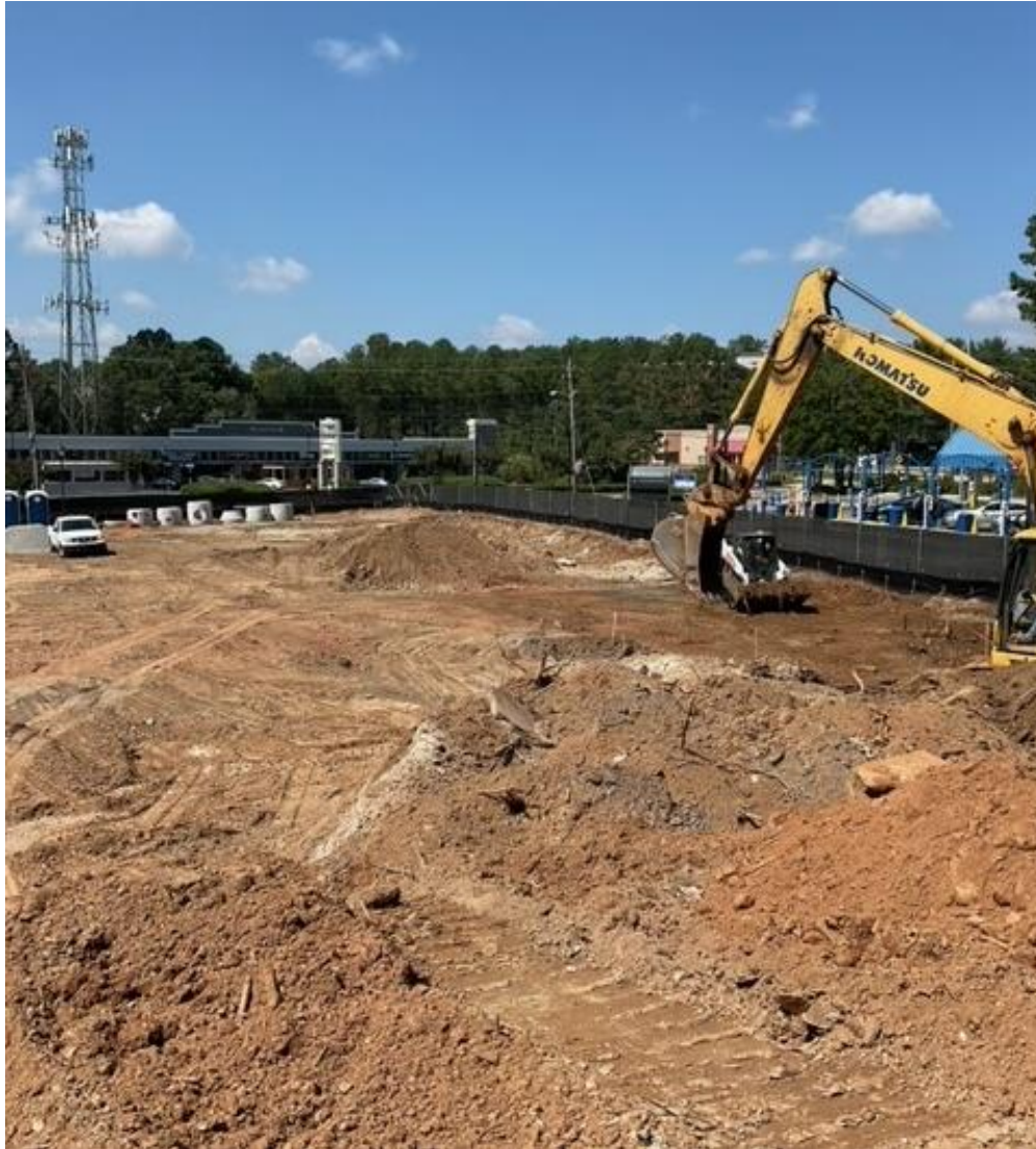
Continued Building Pad Preparations
