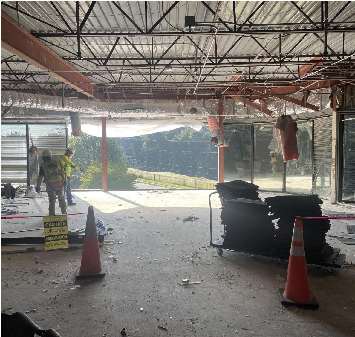
Demo of Existing Conditions
