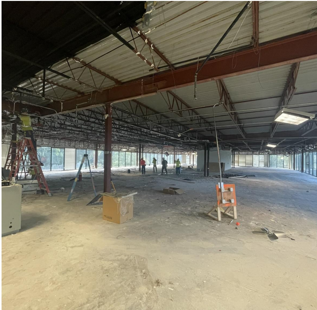
Demo of Existing Conditions
