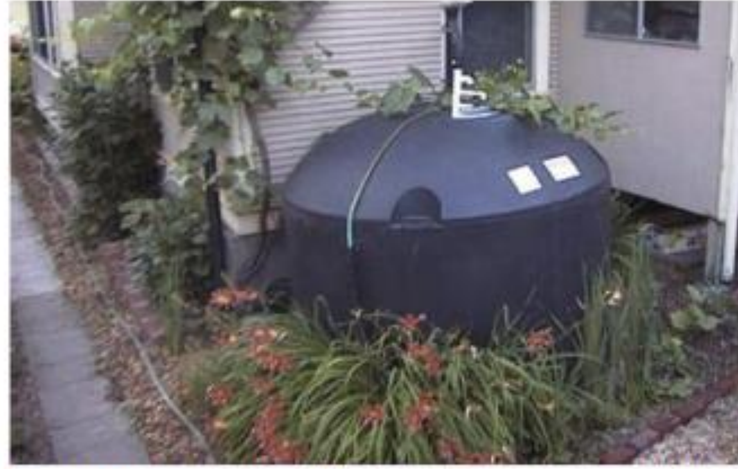
Figure 1 | 1500 gallon cistern (LID Urban Design Tools via City of Atlanta)
