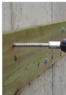
Ledger Installation
