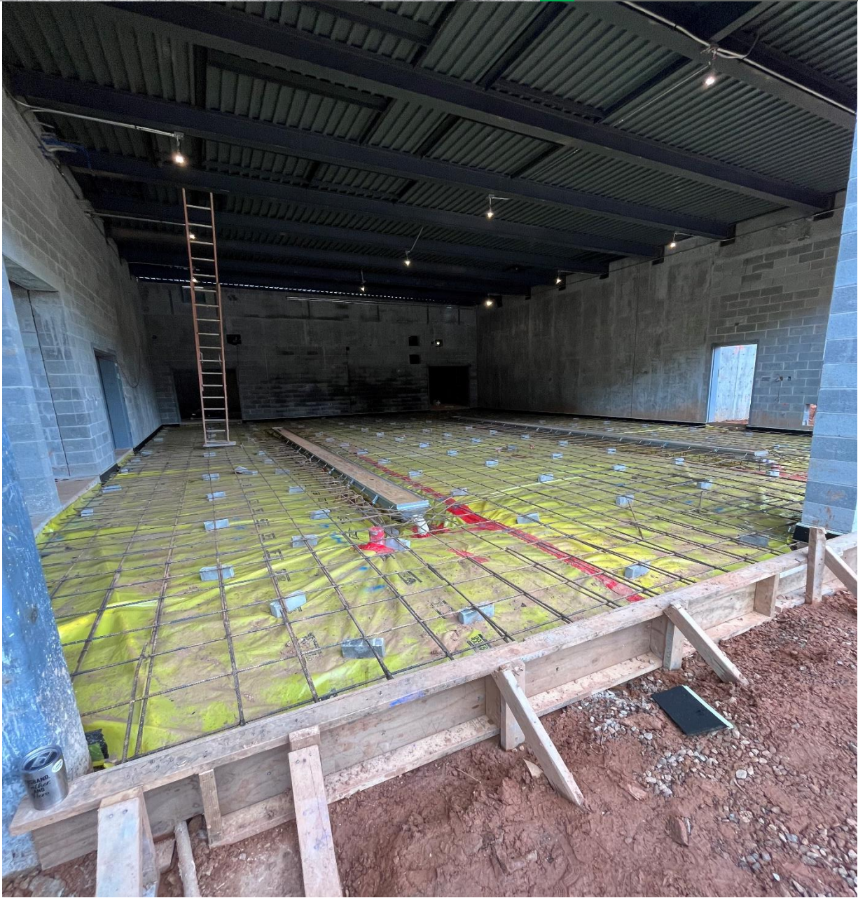
Completed Concrete Prep at Apparatus Bay.
