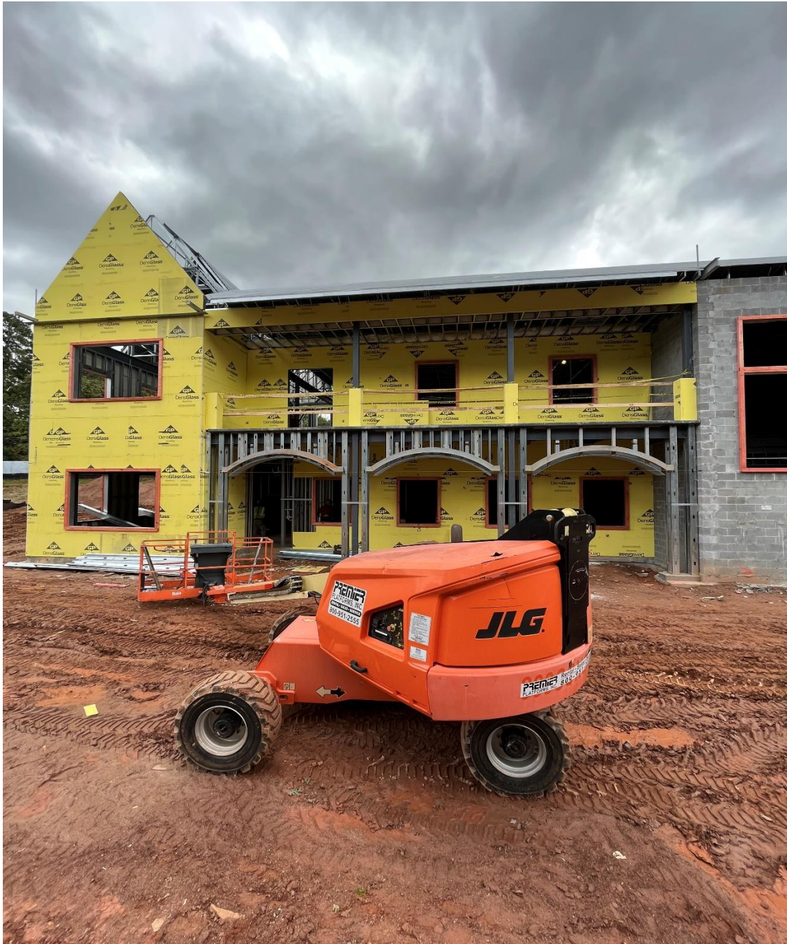
Completed Exterior Sheathing on First and Second Floor.
