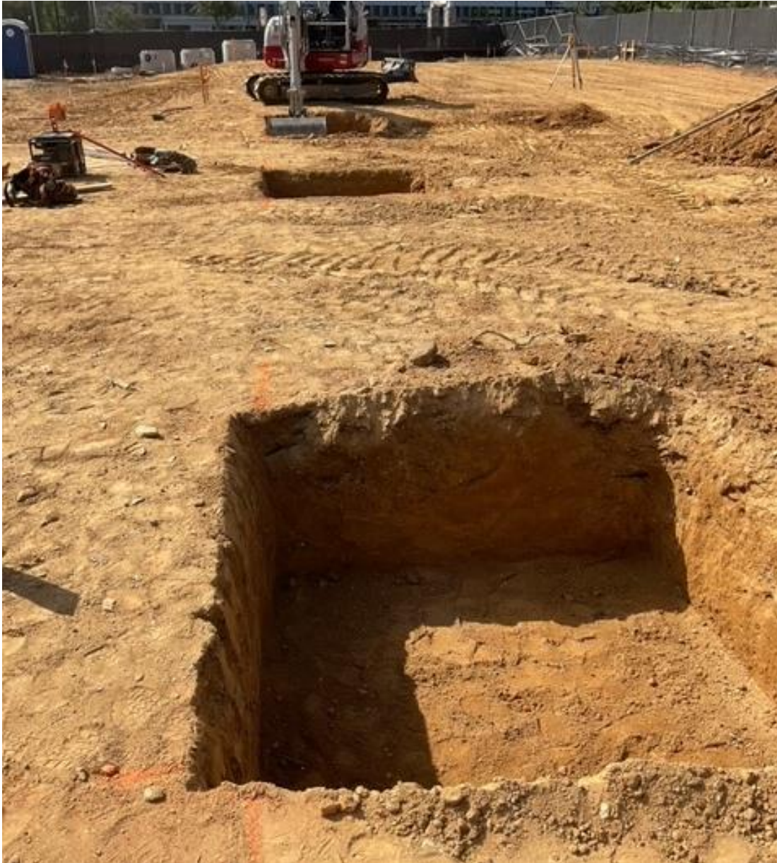
Preparations For The Footings
