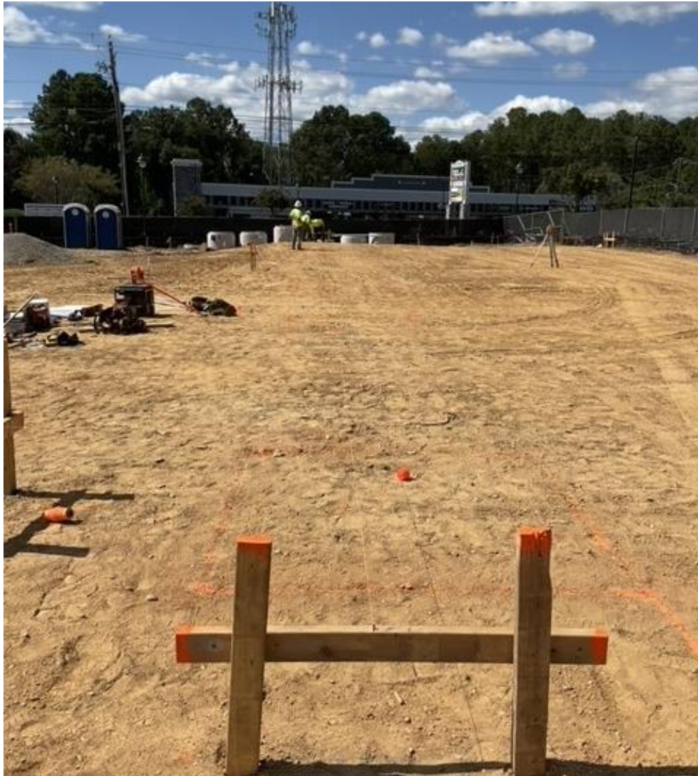
Continued Building Pad Preparations
