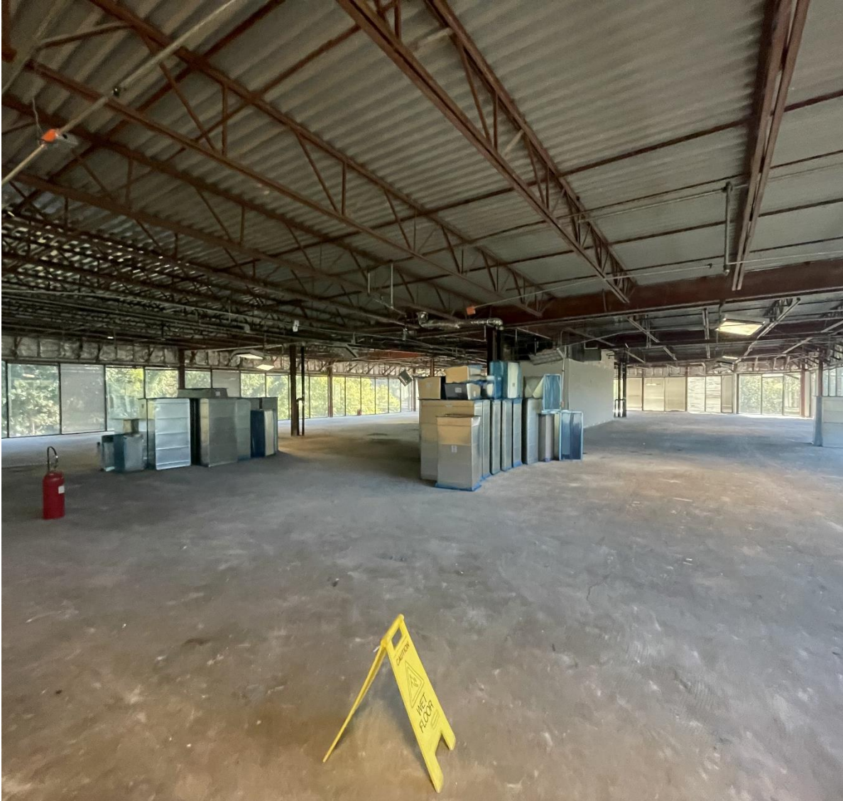
Staging Material for OH Mechanical Rough
