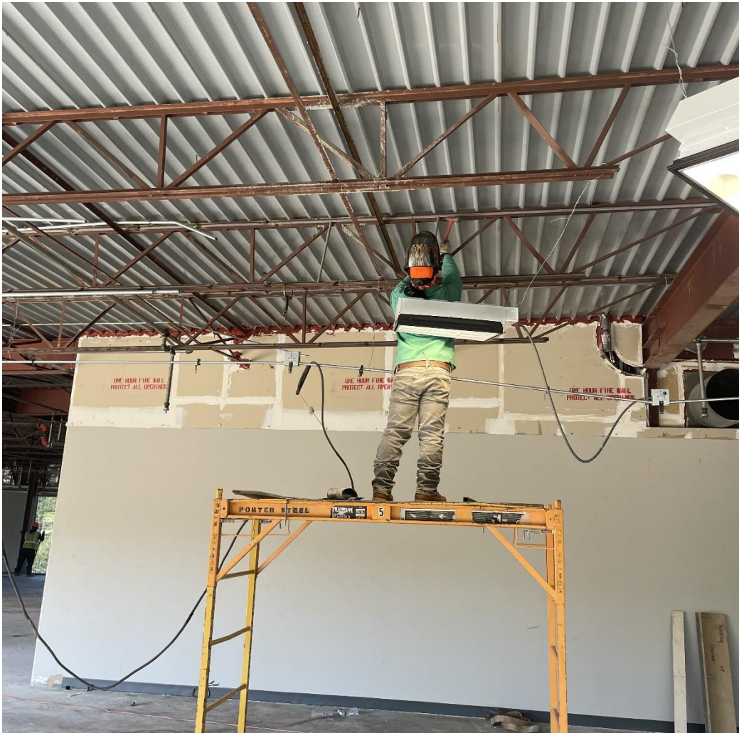
Begin joist augmentation
