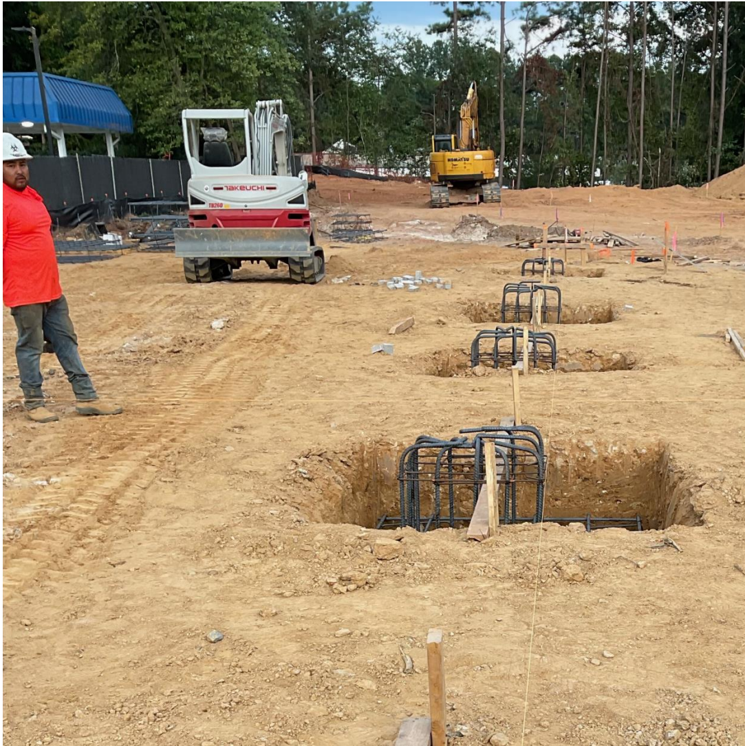
Begin Pouring Footings and Piers
