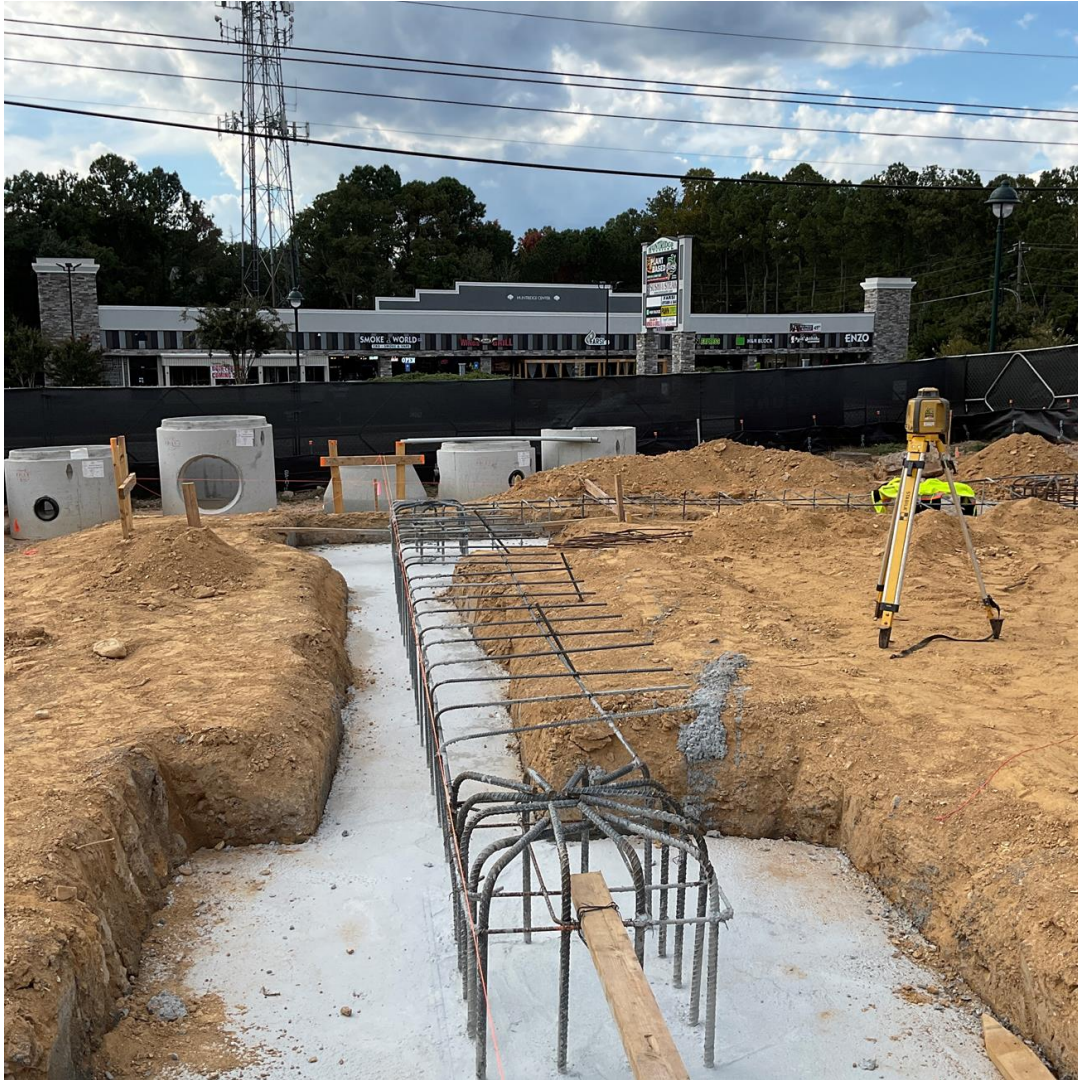
Finishing Pouring Building Footers
