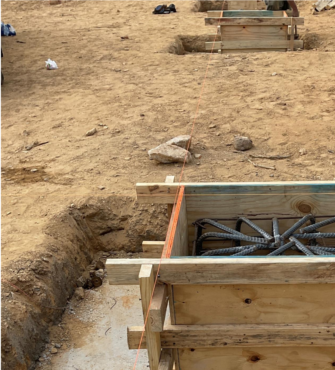
Prep for pouring piers
