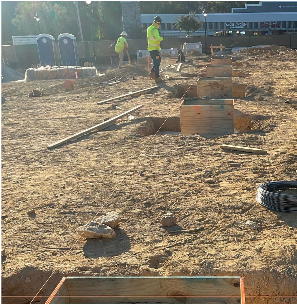
Prep for pouring piers
