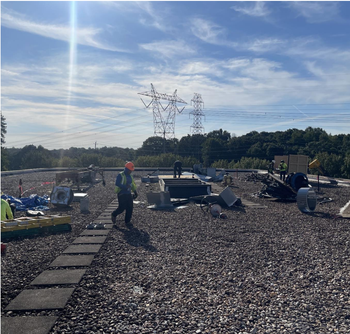
Demolition Of Existing Rooftop Equipment
