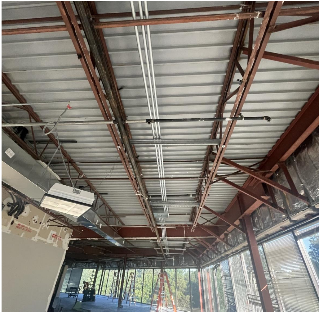
Complete Joist Augmentation on Level 3
