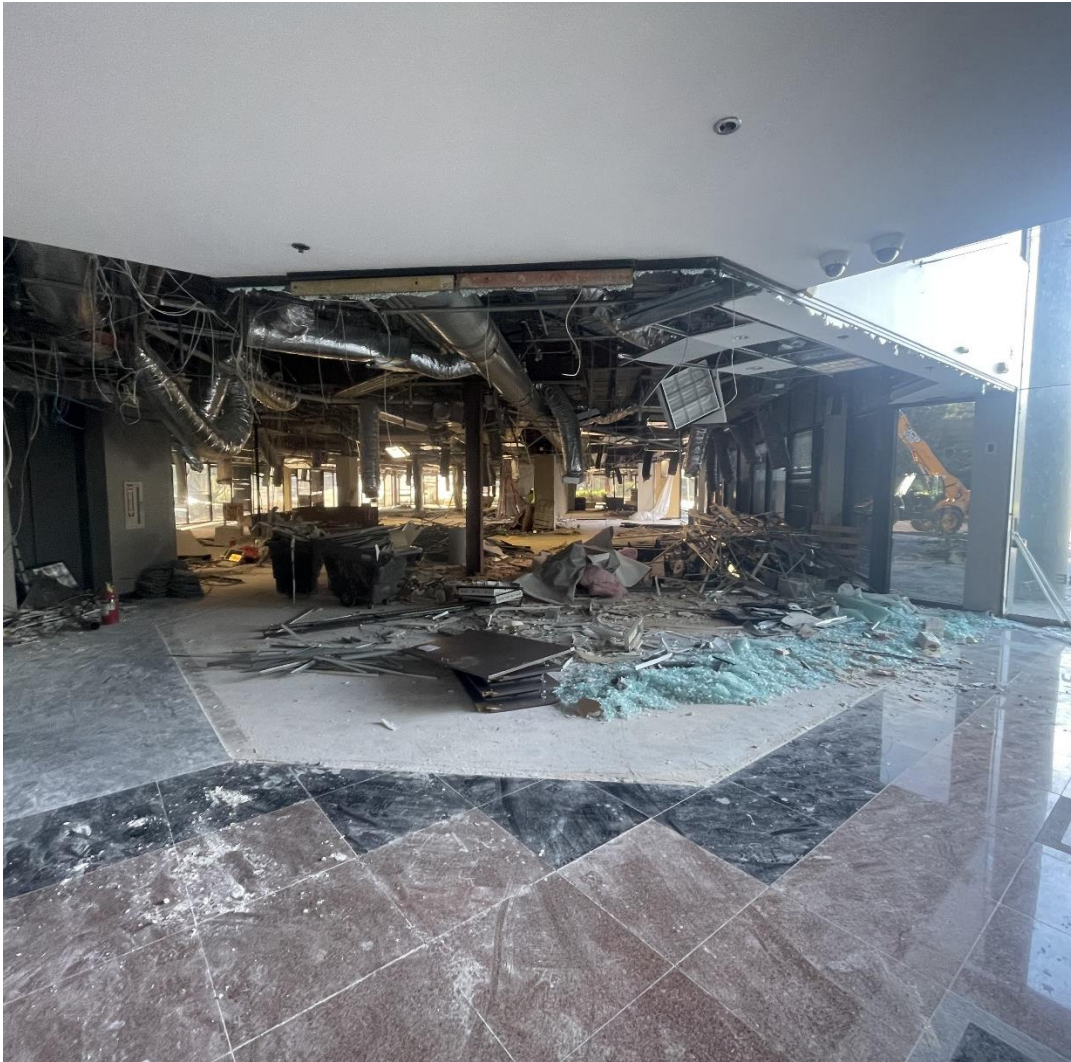
Demolition Of Interior Walls/Ceilings/Flooring On Level 1
