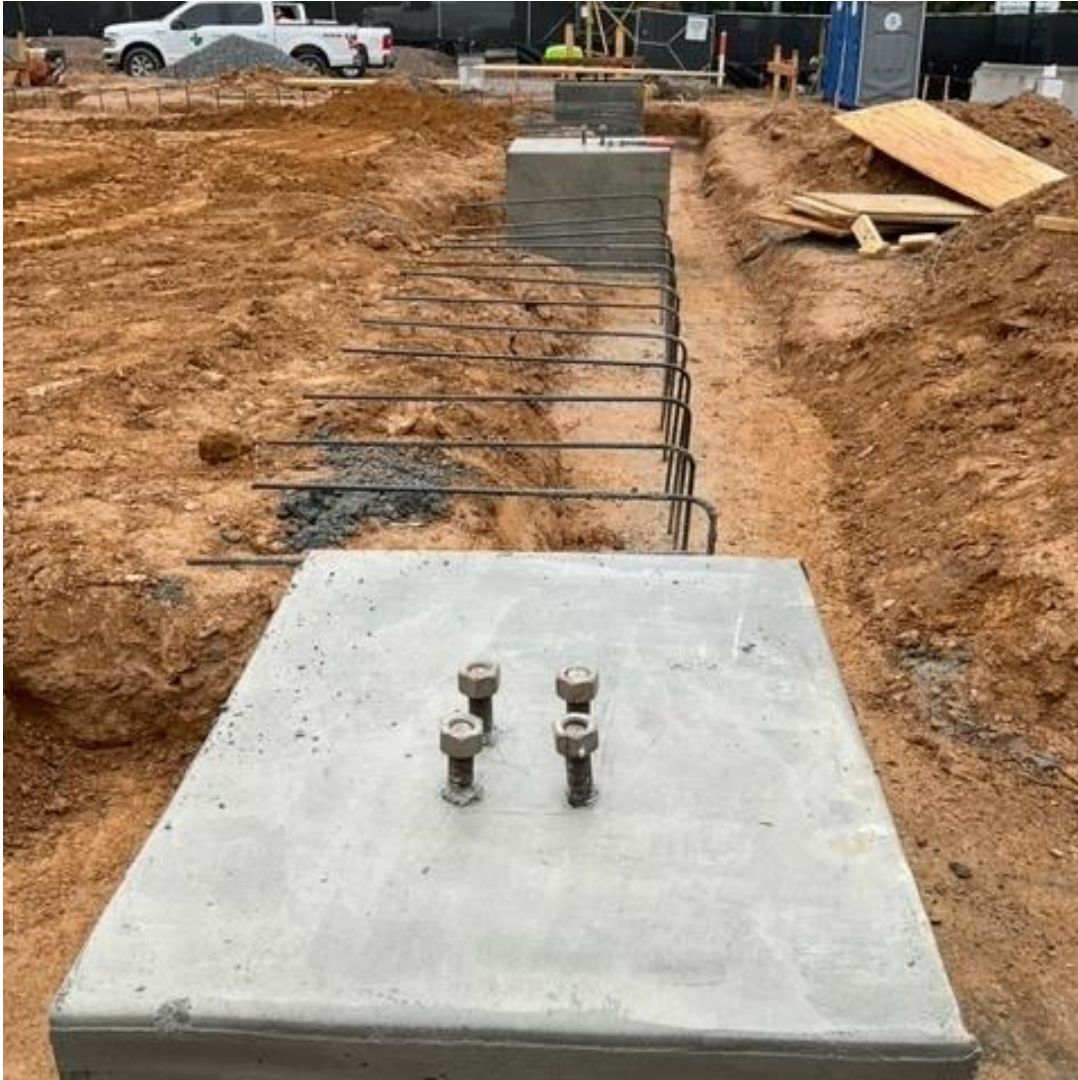
Finish Pouring Footings and Piers
