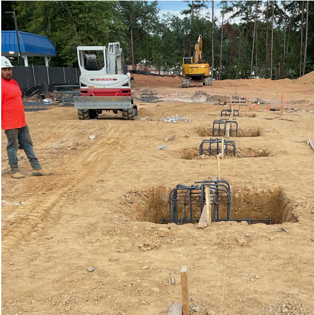
Pouring Footings and Piers
