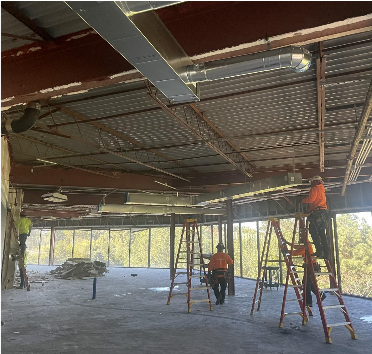
Overhead MEP Rough-in On Level 3
