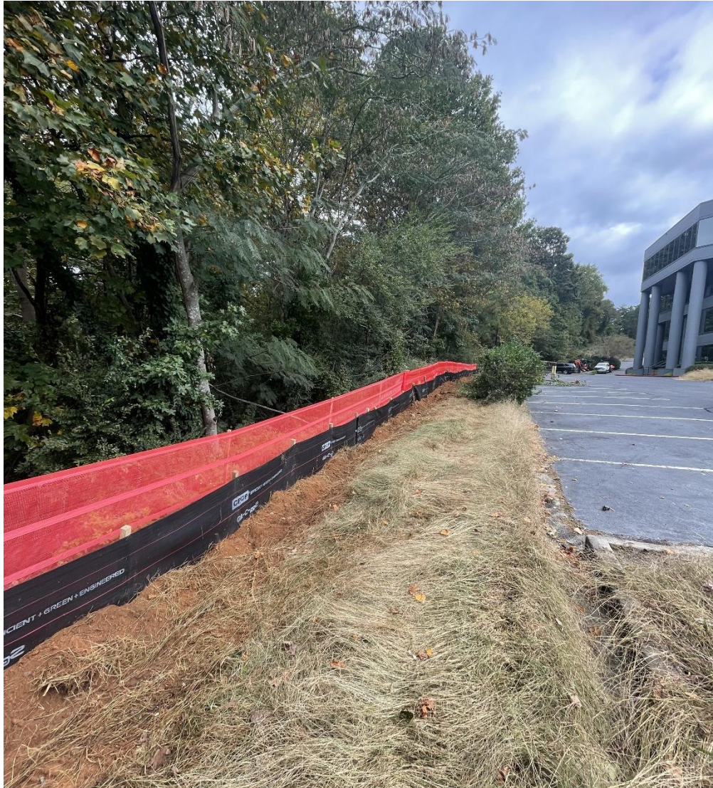
Clearing And Grubbing Of The Site
