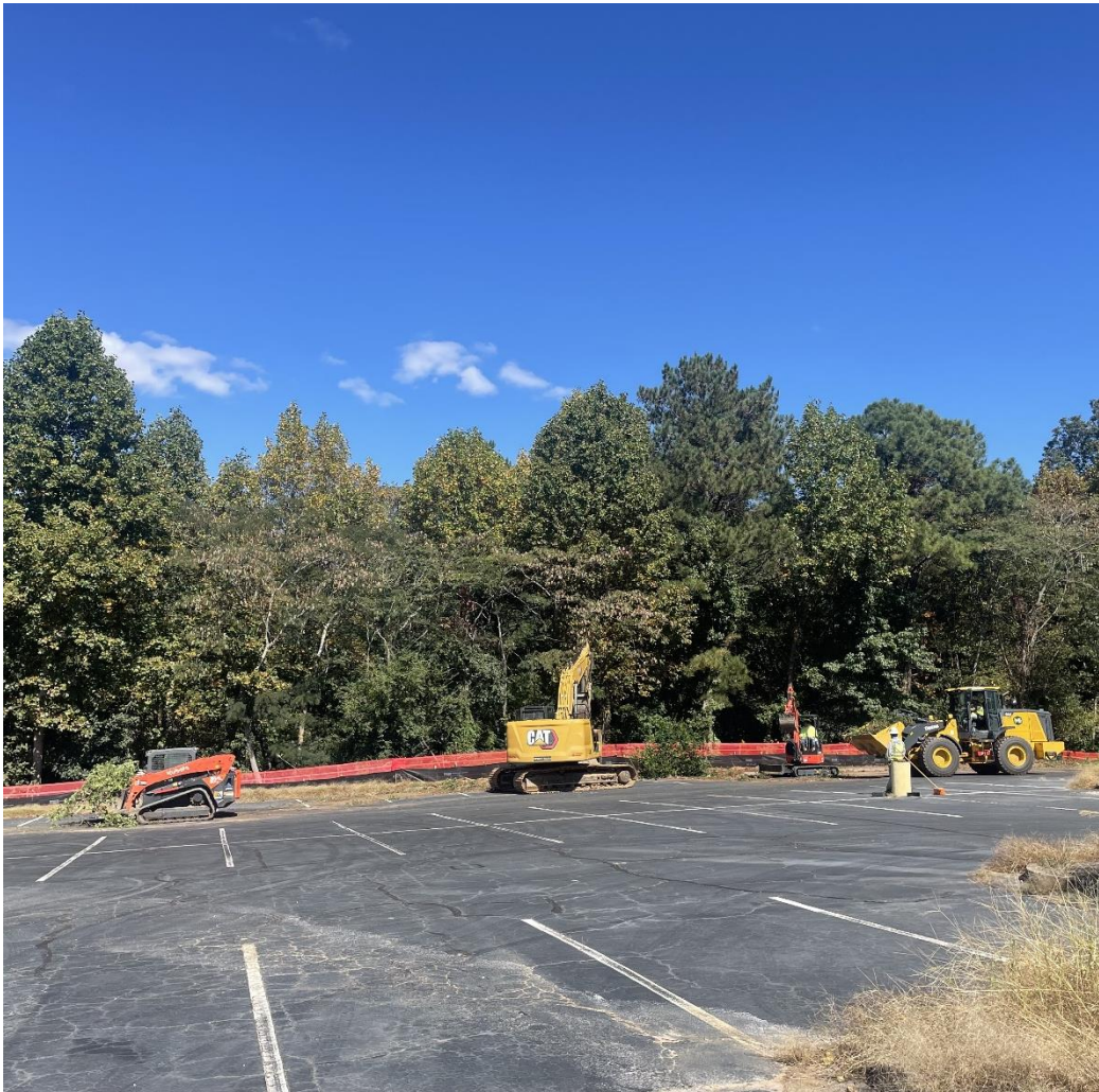
Clearing And Grubbing Of The Site
