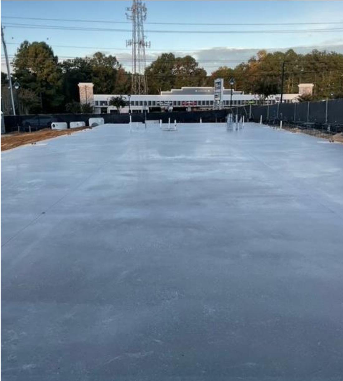
Completed Pouring SOG
